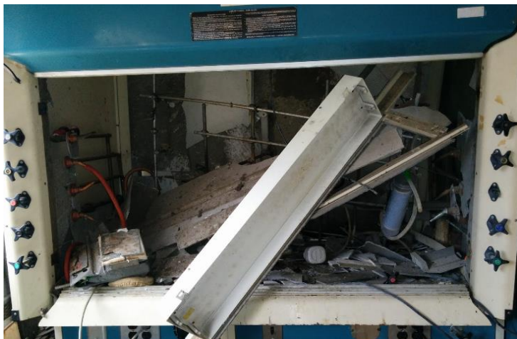
Fume hood after the explosion
