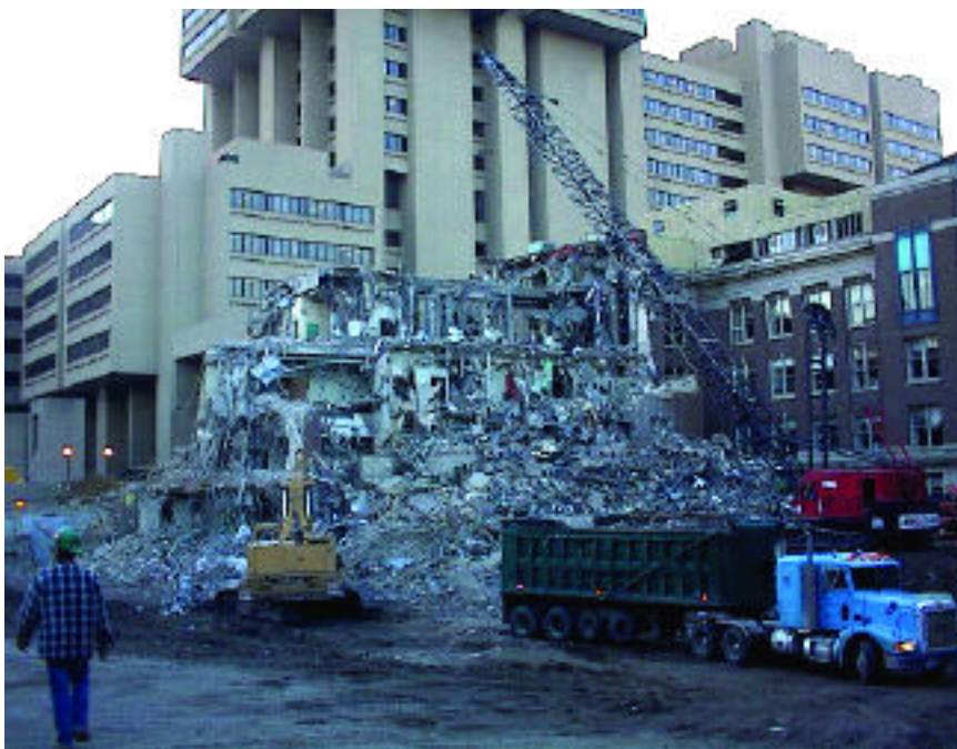
This demolition project near 10 health-care buildings on the University of Minnesota campus was preceded by an extensive ICRA.
