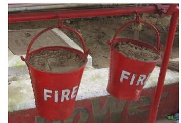
Figure 2: Buckets of Sand for Extinguishing a Fire
